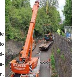
The Grade II-listed cast iron footbridge was taken away for repair after Bristol City Council closed the 'unsafe and unstable' bridge in 2015. It had sustained damage to its underside after twice being hit by vehicles. The bridge has been raised 1 metre higher and steps installed at either end. The £1.1m restoration project was funded by
